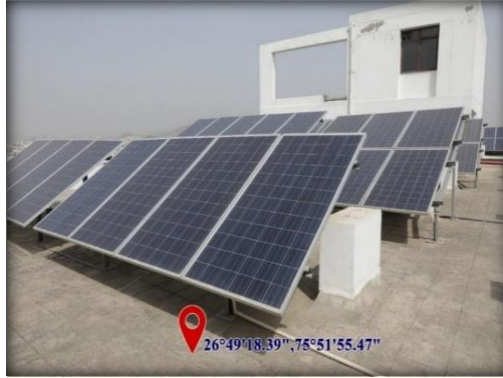
400 kW Rooftop Solar PV Plant
