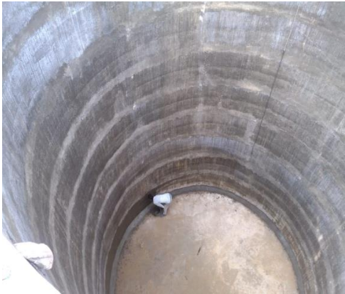
Rainwater Harvesting System (4.5 Lac Liters)
