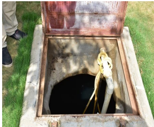
Rainwater Harvesting System (4.5 Lac Liters)
