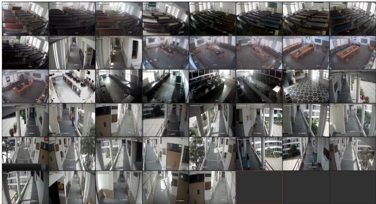
CCTV Coverage area
