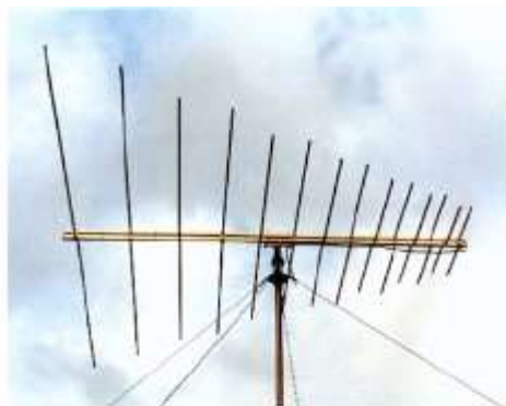
A typical log-periodic antenna pattern
