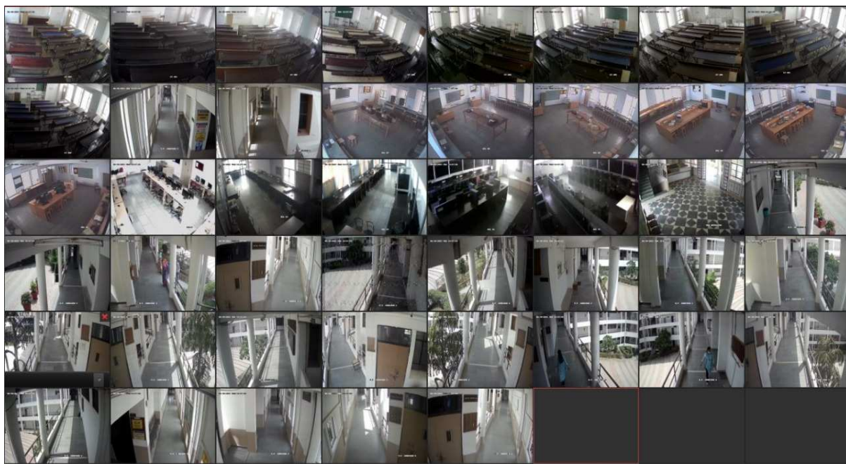
CCTV Coverage area
