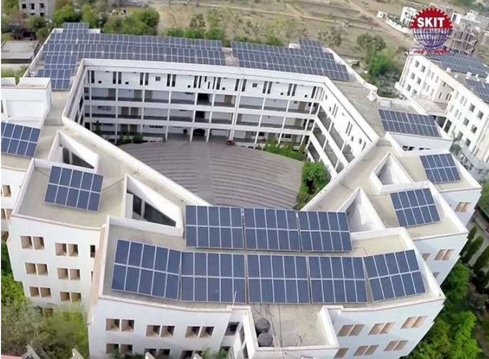
Aerial view of solar power plant
