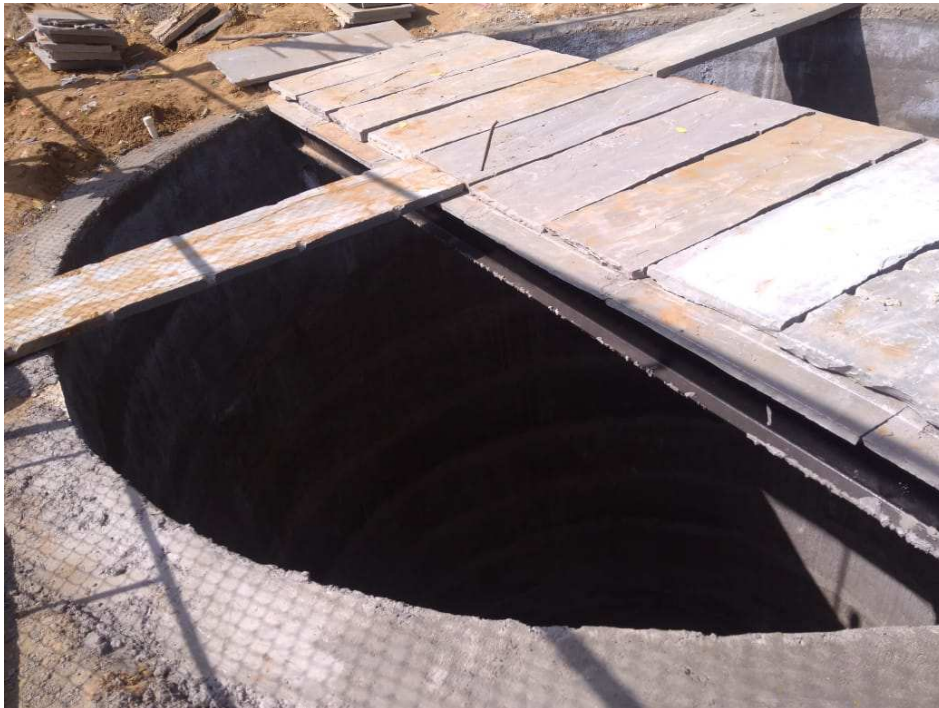
Water Harvesting System: Construction of Underground Tank
