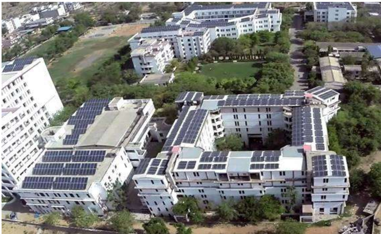
Photo- Solar Power Plant, SKITM&G (400 kW Rooftop)
