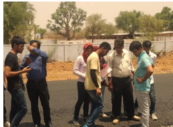
Evaluation of newly constructed road
