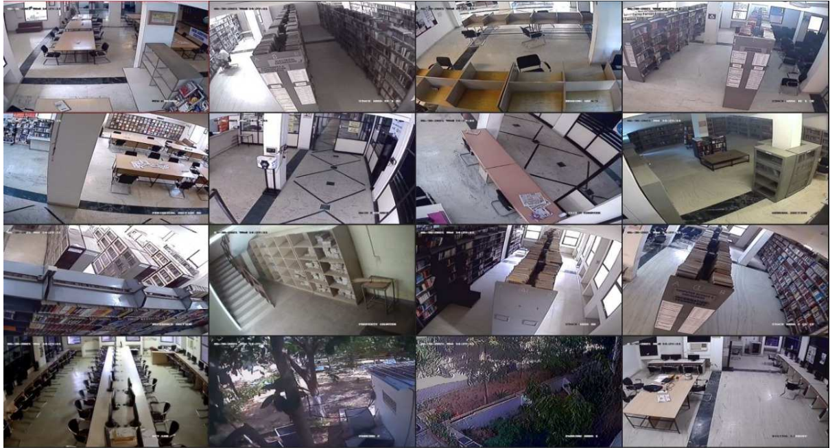
CCTV Coverage area
