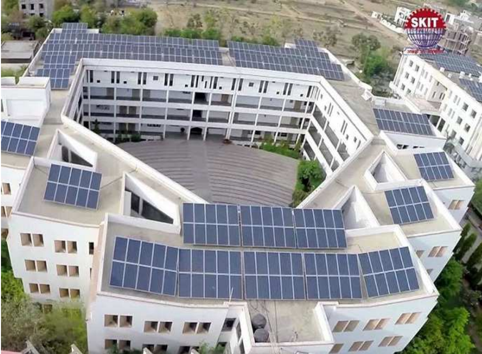
Aerial view of solar power plant
