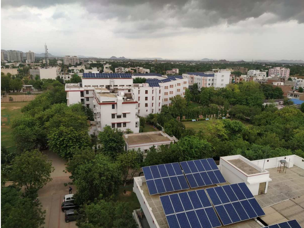
Photograph of Solar Power Plant
