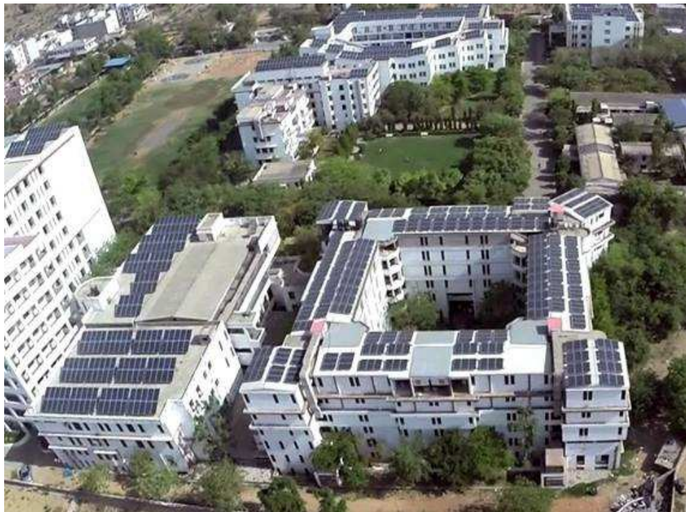
Aerial view of solar power plant
