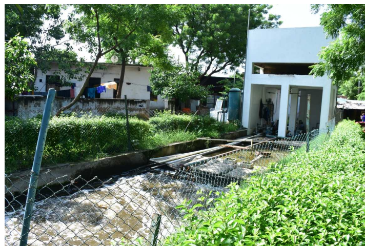
Sewage Treatment Plant
