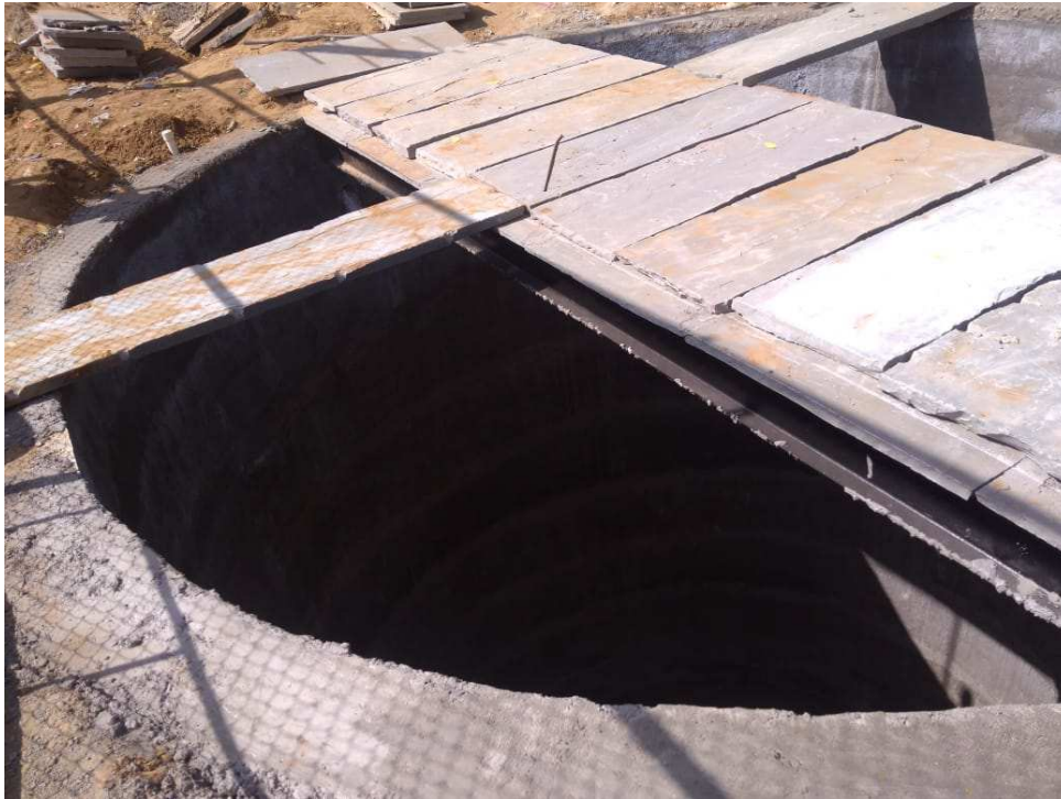
Water Harvesting System: Construction of Underground Tank
