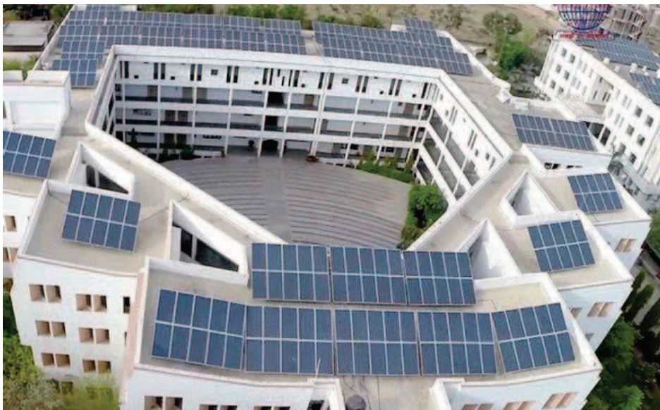
Installed 400KW Capacity of Solar at Rooftop of SKIT
