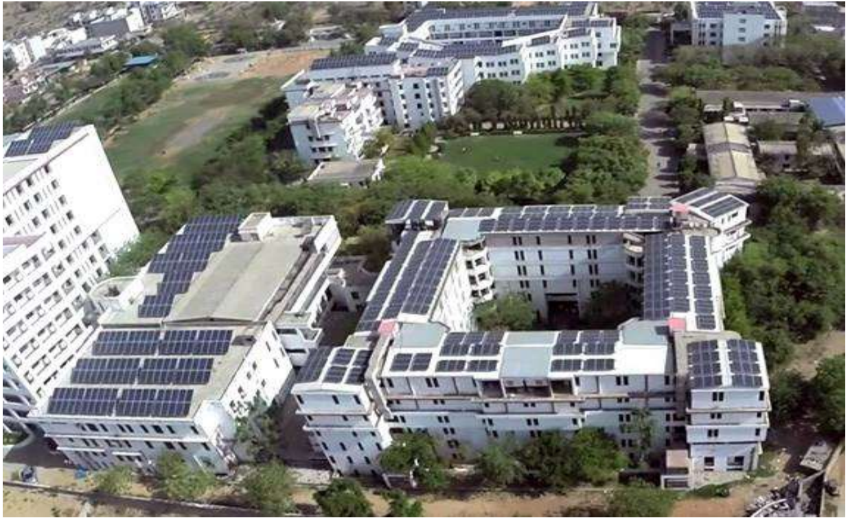
Photo- Solar Power Plant, SKITM&G (400 kW Rooftop)
