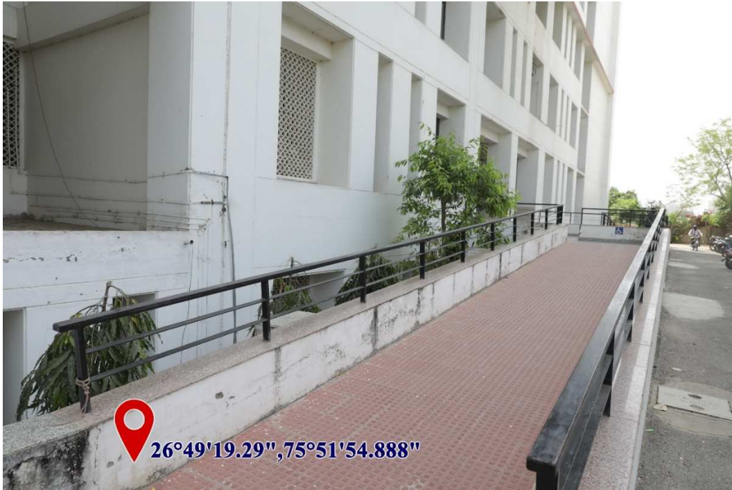
Ramp for easy access to Classrooms & Labs
