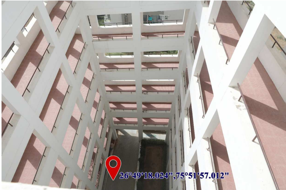
Ramp for easy access to Classrooms & Labs
