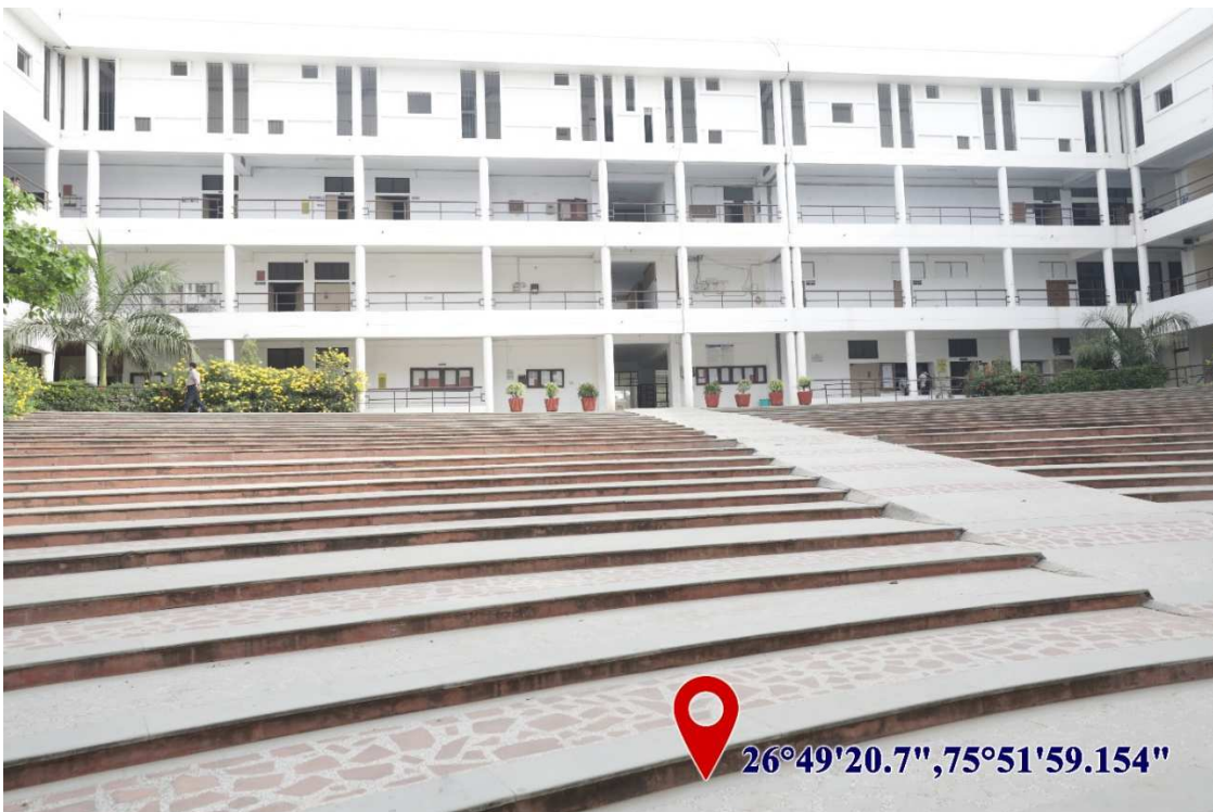
Ramp for easy access to Classrooms & Labs
